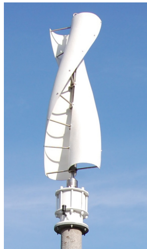
ABOVE: Vertical axis wind generators may vary in appearance. Blades that present a solid appearance (such as the left image) are encouraged.
